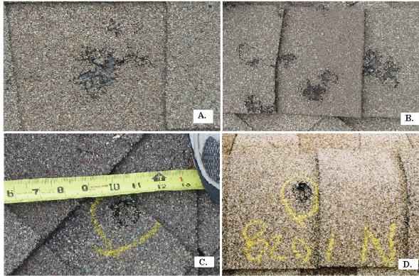
Figure 10. A) Location 21-Hail impact puncture in laminated shingle that overlaid wood shingles; B) Location 25-Multiple hail impact-caused bruises in hip shingles; C) Location 72-Hail-caused bruise in unsupported valley shingle; D) Location 82-Hail-caused puncture of unsupported region of high-profile ridge shingle.
