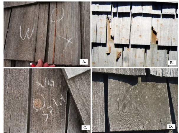
Figure 13. A) Location 105-Gray split from weathering (left) and fresh split from hail impact (right); B) Location 86-Shake pieces broken off by hail impact; C) Location 105-Large hail impact without a split; D) Location 15-Small impact marks on shake surface (no hail impact damage).
