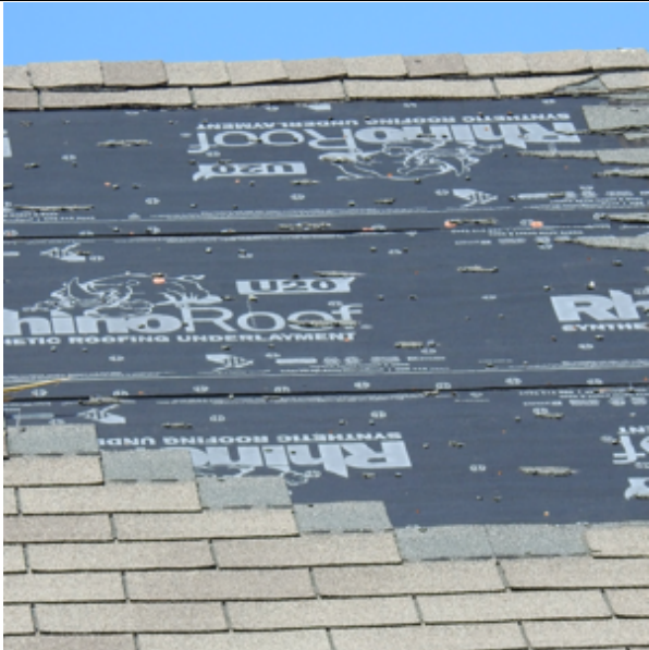
Photo 157: Fully intact underlayment
