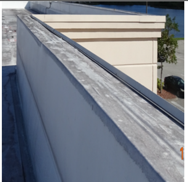
Photo 20: Coping that is undamaged.
