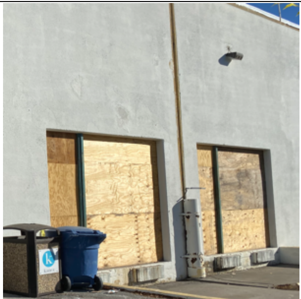
Photo 62: Primary source of roof damage, door failure pressurizing the roof.
