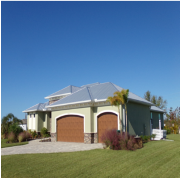
Photo 85: Through fastened metal Roof Survivor of 130 mph winds. Open terrain.
