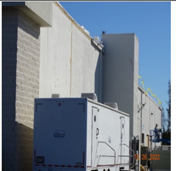
Photo 65: Missing gutters
