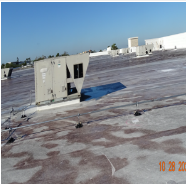
Photo 21: Overview of the CASE STUDY 6 roof.
