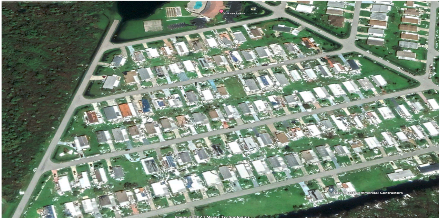
Figure 1. The view is from Google Earth on 9/29/2022 and shows significant roof and structure damage. This area of modular homes was developed between the years 1994 and 1998. This subdivision was just north of Rt 776 and in the highest wind area with projected 130 mph winds.
