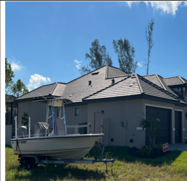
Photo 115: SW 39 th Ave Winds of 110 mph. No damage observed
