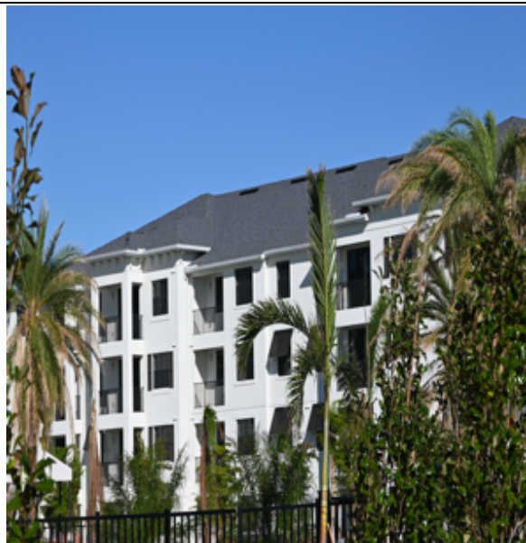
Photo 141: New construction and asphalt shingles
