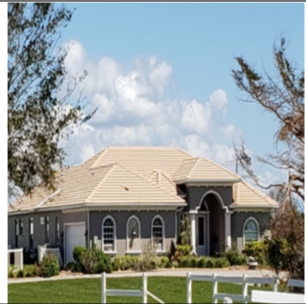
Photos 123 & 124: These roofs appeared undamaged despite 130 mph winds and are in very flat terrain with few obstacles i.e., likely Class C wind exposure.
