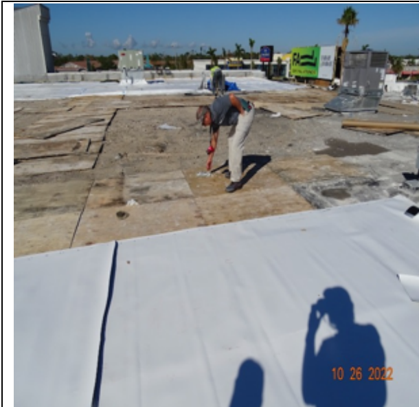
Photo 64: Temporary fastening to deck
