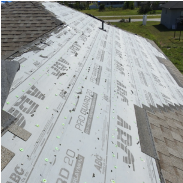
Photo 156: Although the shingles were missing, the underlayment in most cases kept the building dry.
