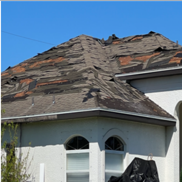
Photo 159: Some damaged underlayment was observed on this older asphalt shingle roof.
