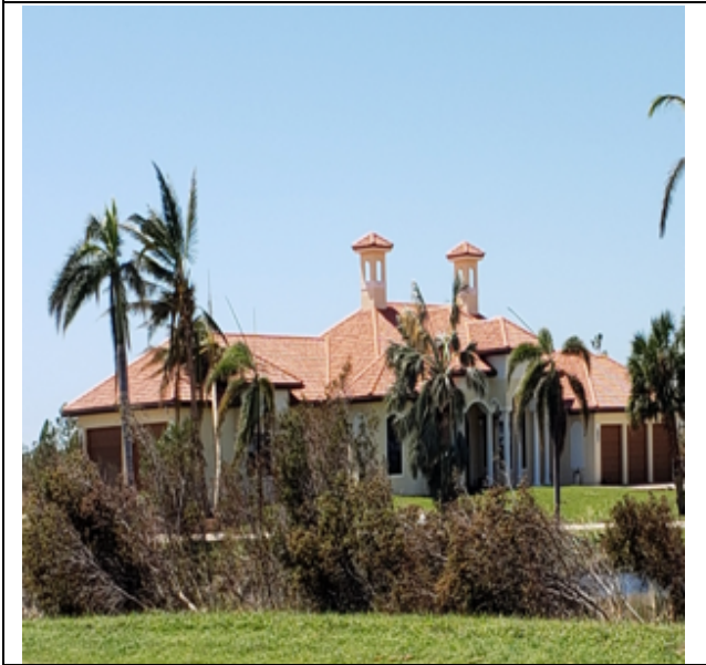
Photos 123 & 124: These roofs appeared undamaged despite 130 mph winds and are in very flat terrain with few obstacles i.e., likely Class C wind exposure.
