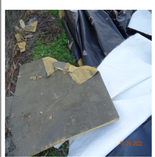
Photo 3: This was insulation/cover board retrofit over a CWF deck.
