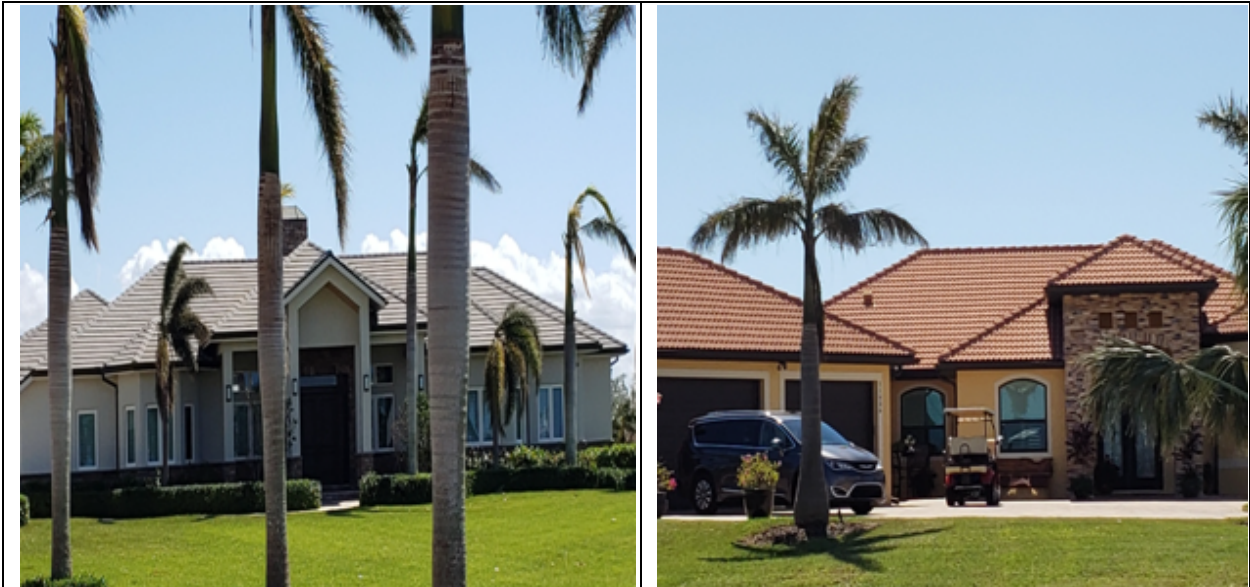
Photos 125 & 126: These roofs appeared undamaged despite Class C wind exposure and 130 mph winds so neatly cleaned up.
