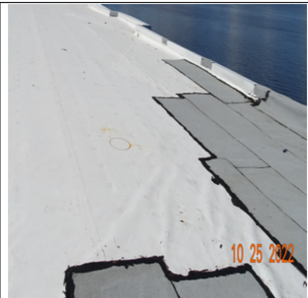
Photo 26: Emergency (temporary) repairs to adjacent building.
