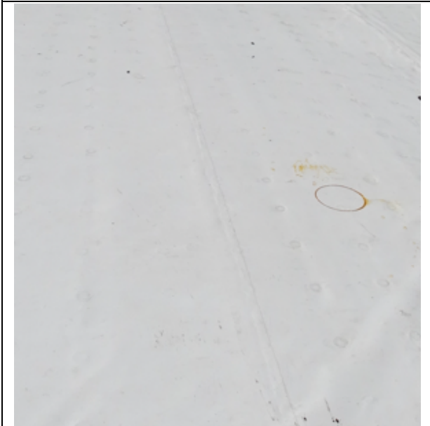
Photo 27: A tight fastener pattern is visible securing this membrane.
