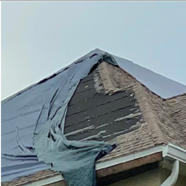
Photo 158: Asphalt impregnated felt underlayment appeared intact.
