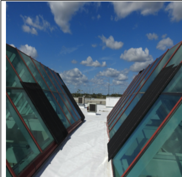
Photo 50: Damaged Skylights
