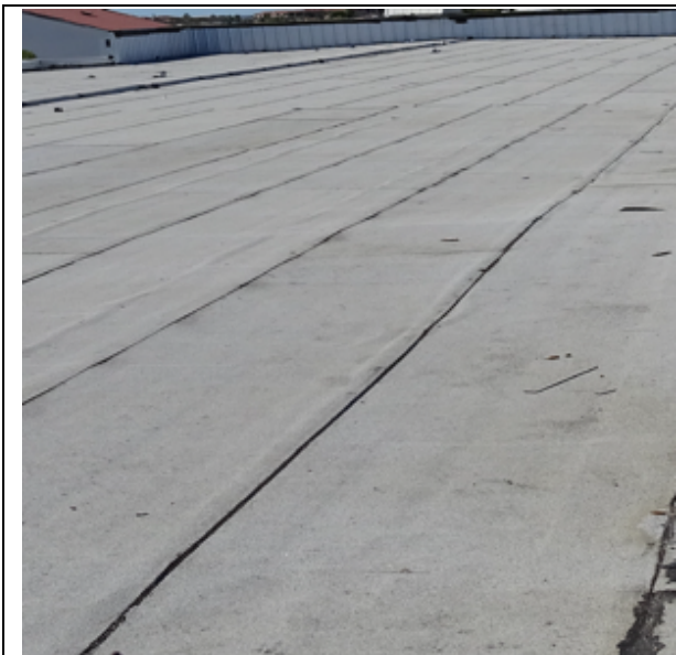
Photo 25: Temporary roof over entire building.
