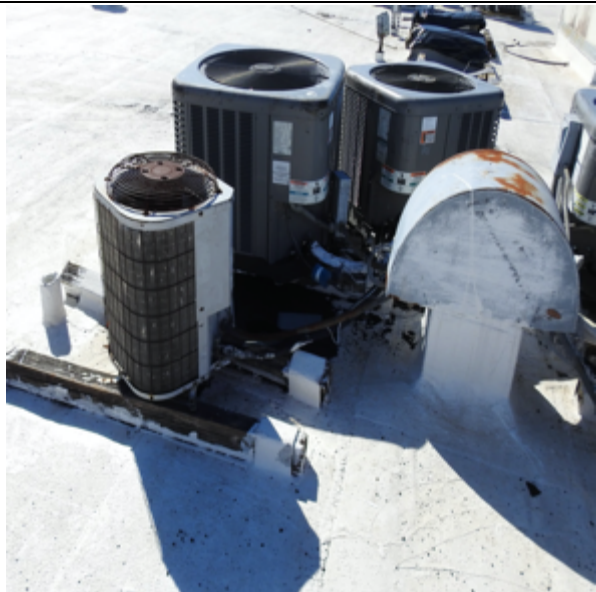
Photo 45: Displaced AHU
