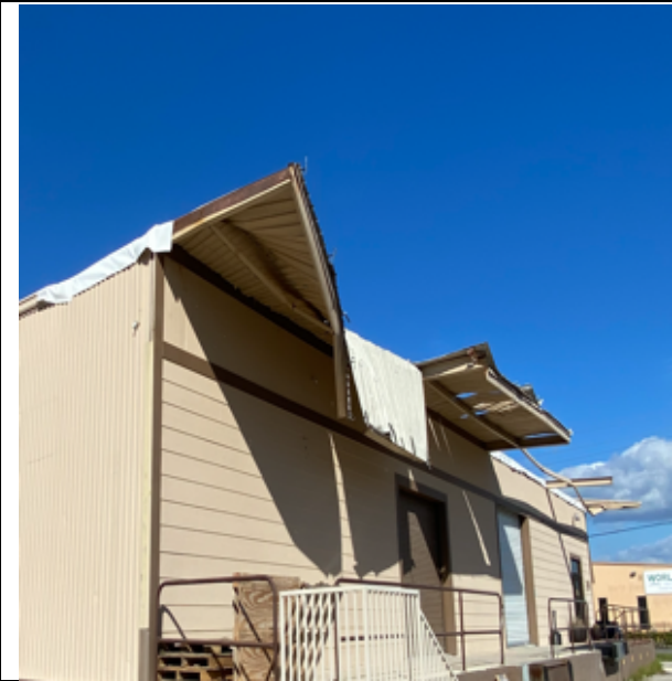
Photo 78: Overhang damage
