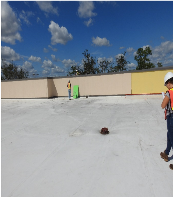
Photo: 55a the rest of the roof had 5ft parapets and was not damaged
