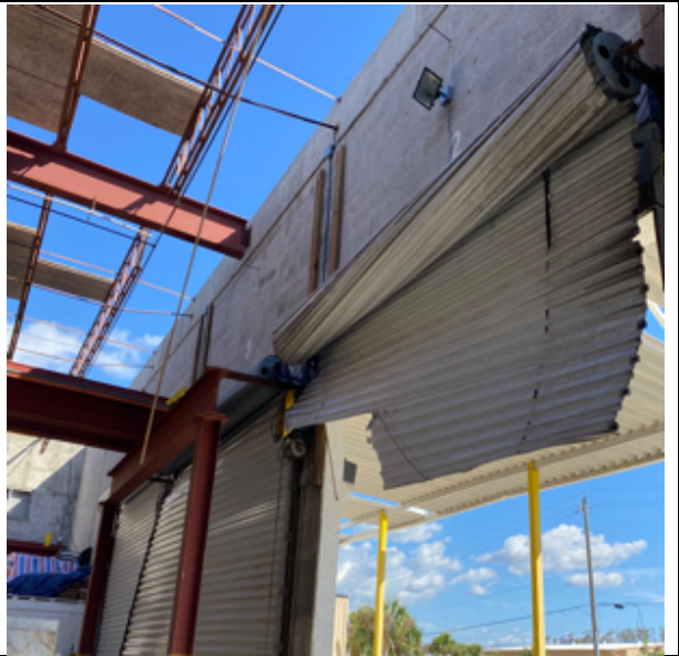
Photo 2: Stone Warehouse - Extensive loss of CWF roof deck.
