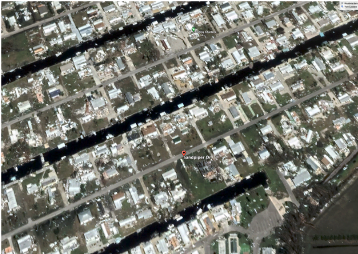
Figure 6: This neighborhood on Pine Island was mostly built between 1985 and 1995. It had significant damage from 120 mph winds and storm surge.
