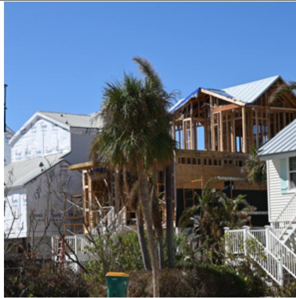
Photo 155: Appears to be siding and roof damage
