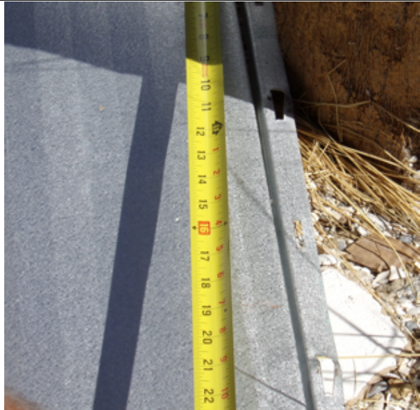
Photo 97: This roof had seams 16 O.C. and fastening 10" O.C.
