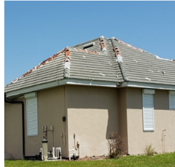
Photo 107: Lack of full foam contact at the hip and allowed ridge tiles to become detached, becoming windblown projectiles, and further damaging the roof.
