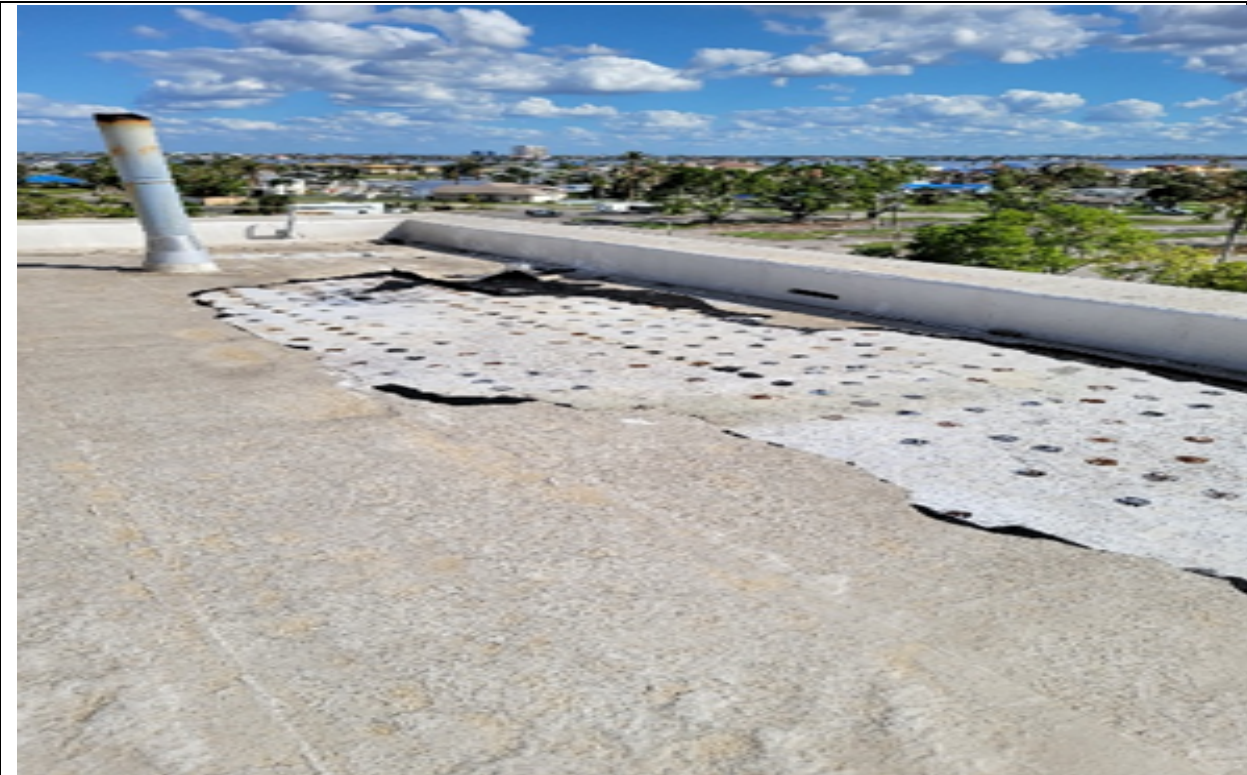
Photo 45a : Membrane peeling exposing the lightweight insulating concrete and fasteners and plates
