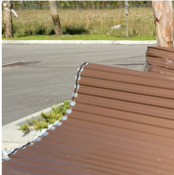
Photo 163: Missing overhead (roll-up) door
