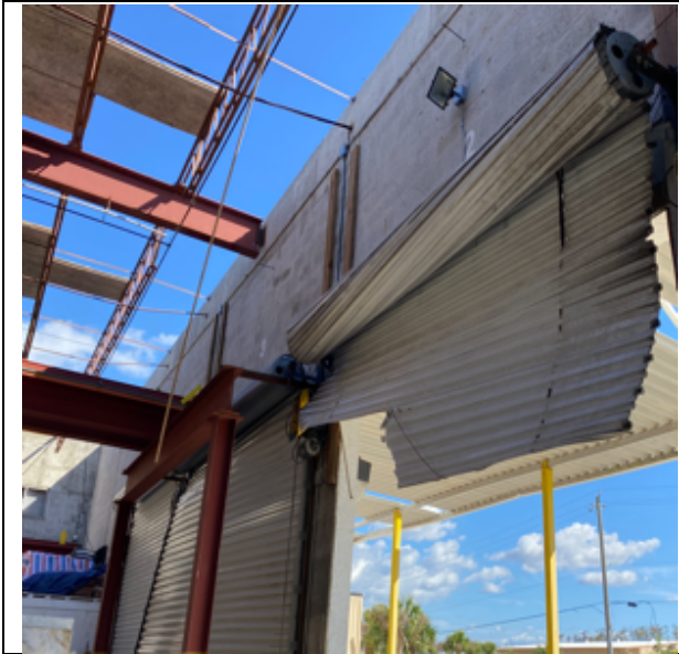
Photo 1: Stone Warehouse - One photo tells a lot. Overhead door failure caused a pressurized building, leading to blow off of cementitious wood fiber deck & membrane.
