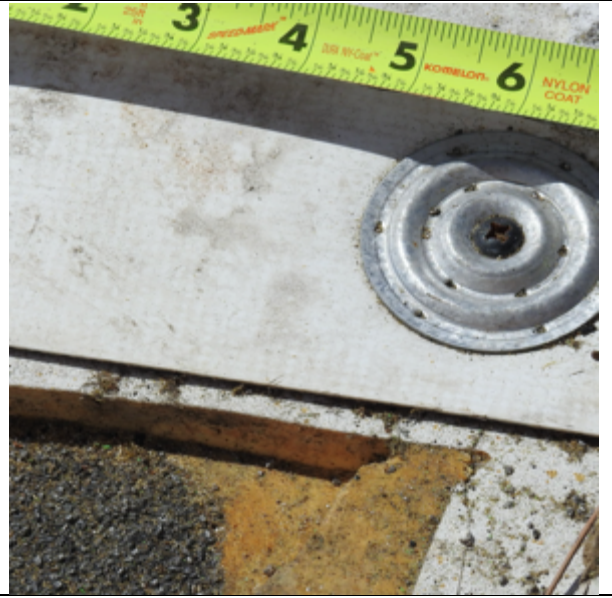
Photo 55: Initial fastening over BUR roof.
