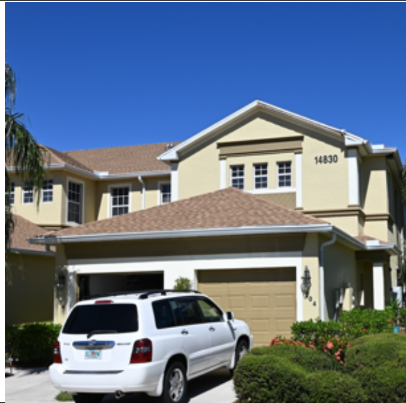
Photo 143: Many asphalt roofs in this area were intact. This neighborhood was built in 2005 and it appears to have been reroofed about seven years prior to the hurricane.
