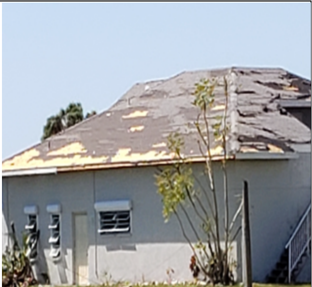
Photo 134: Older asphalt shingles
