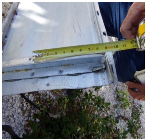
Photo 159: Inadequate fastening
