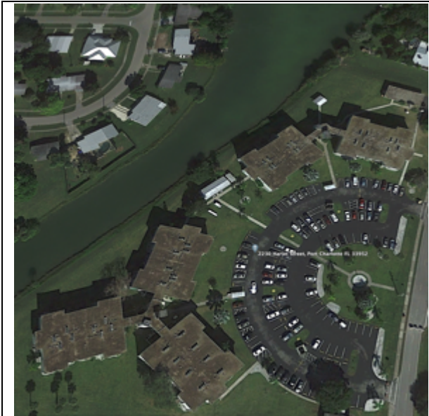
Photo 59: Google earth view (2021) water facing units had most damage
