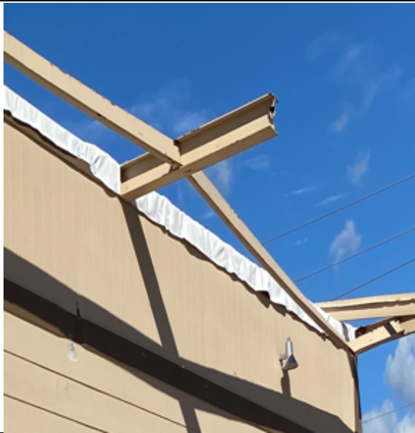
Photo 79: Temporary repairs of metal panel roof
