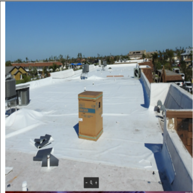
Photo 39: Overview shows ongoing temporary repairs.
