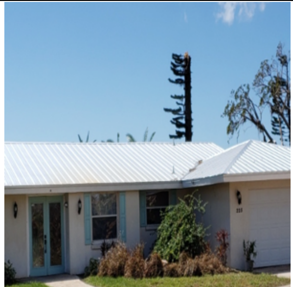
Photo 92: Successful older installation, 120 mph wind
