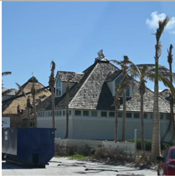
Photo 154: Wood shake roof, being repaired
